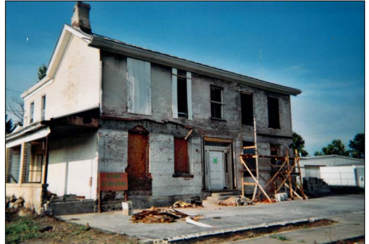
■ The club house building during renovations
