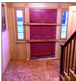
New floor installed in hallway
