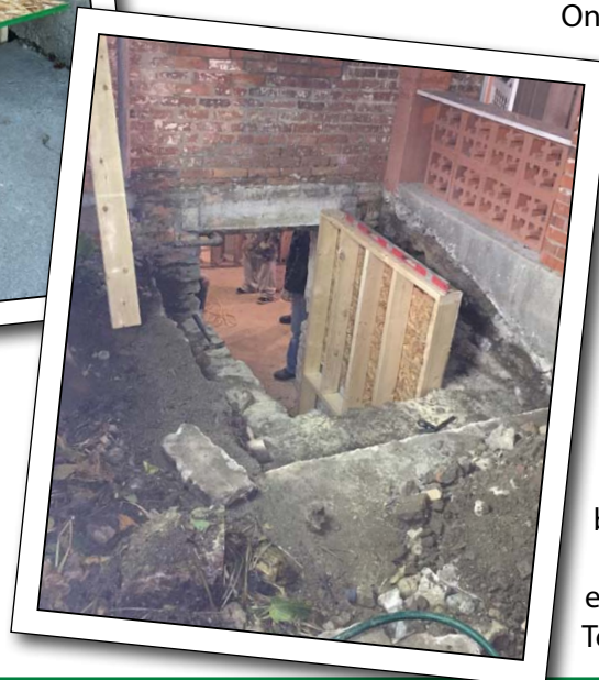
The outside basement door was in bad shape. The door was removed, as were the steps and the concrete around it. A new form was put in place and concrete will be poured. Once the concrete cures, a new steel door will be installed.
