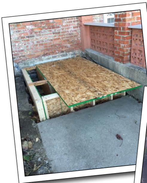
The outside basement door was in bad shape. The door was removed, as were the steps and the concrete around it. A new form was put in place and concrete will be poured. Once the concrete cures, a new steel door will be installed.
