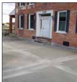
New front concrete pad
