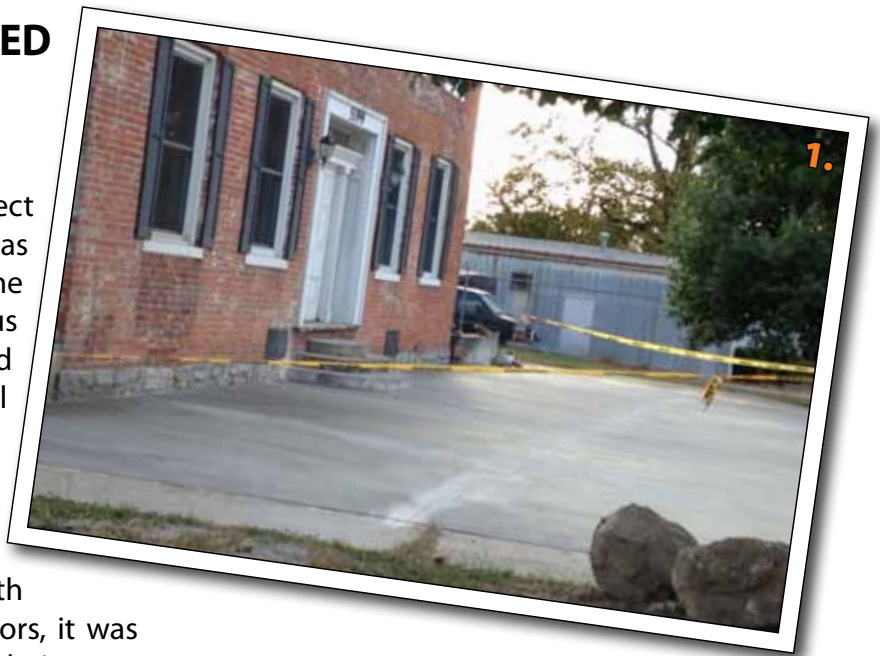
1. New concrete was poured Wednesday, Oct. 14.
