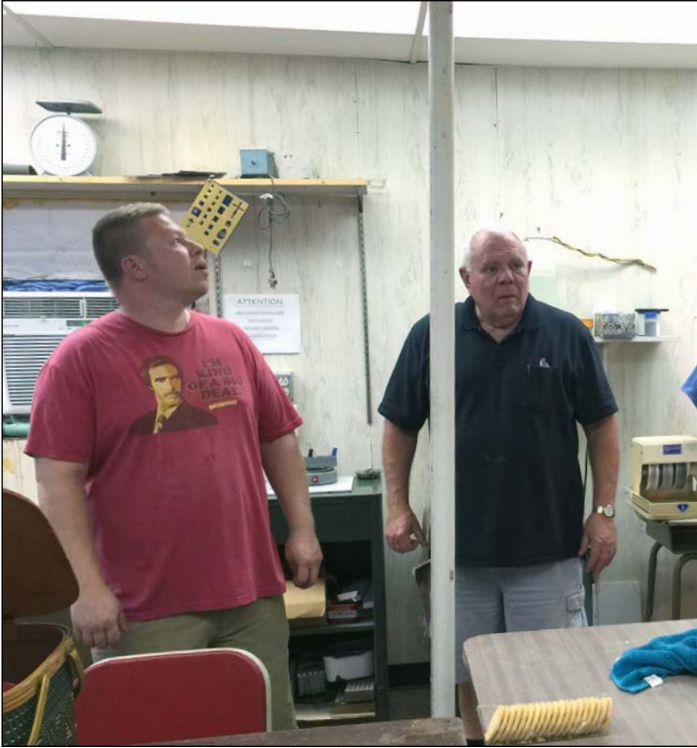
■ The suspended ceiling in the lapidary lab needs some maintenance, and the room itself could use some general cleaning and organizing. No matter your skill level, there will be something for you to help with during the Oct. 22 Club Clean-up Day.
